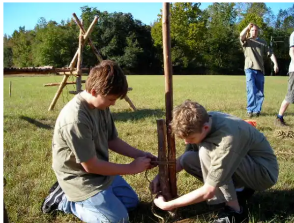
Scouts attach a 6-foot stave to a pioneering stake with two round lashings.
